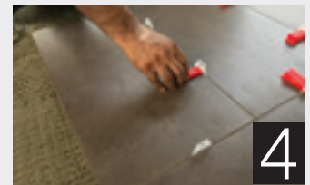
Insert Wedge into the Tile Spacer
