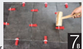
Or simply Remove Wedges with a Mallet
