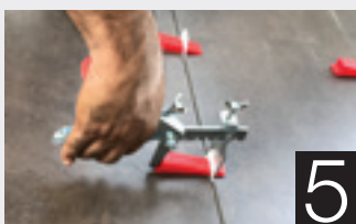
Tighten Wedge using our Special Tool-Plier
