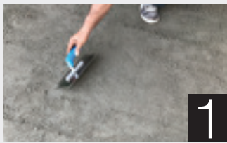
Apply Tile Glue / Cement
